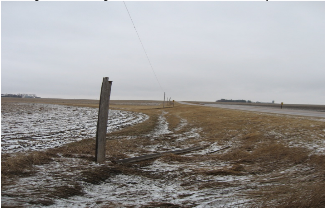
Figure 1: Damaged Power-lines, Osceola County, Iowa
