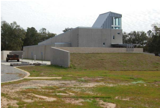
Figure 1. Project 343 East Shelter
