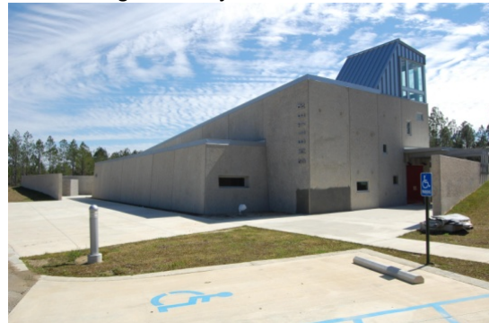
Figure 2. Project 344 West Shelter
