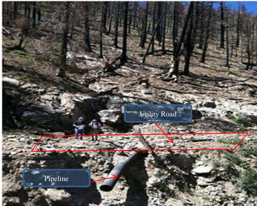
**Figure 1: Damaged pipeline and utility roadway from the declared event.**
