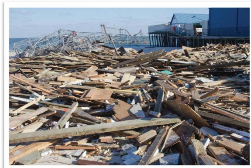
Figure 1: Hurricane Sandy Debris along the Historic Boardwalk in Seaside Heights, New Jersey.
