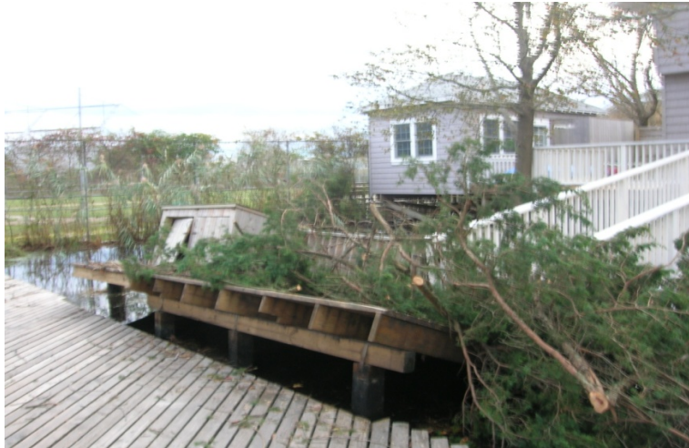
Figure 1. Damaged Boardwalks after Hurricane Sandy
