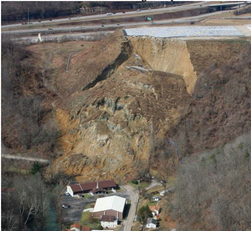
Figure 1: Damage to the Engineered Arresting Structure at Yeager Airport
