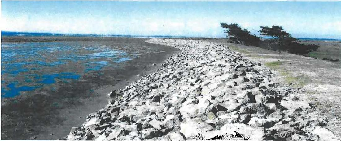
**Figure 1. Levee Riprap Slope Repair**
