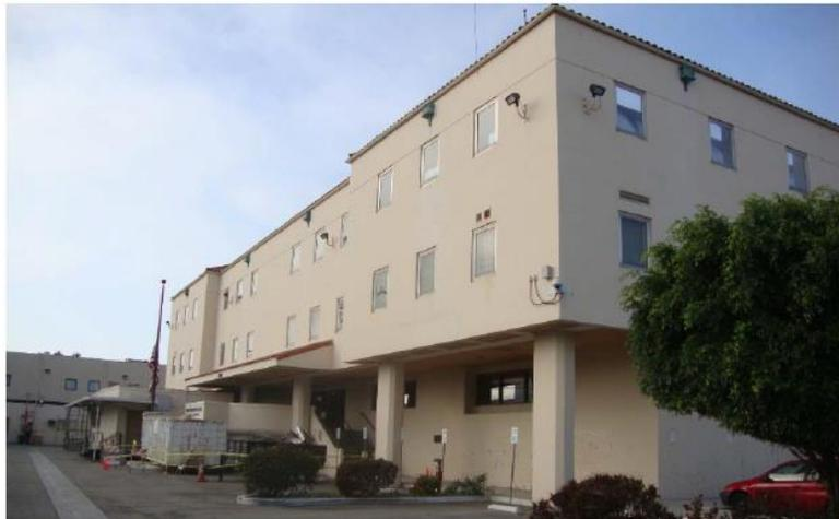
*The San Pedro Service Processing Center was originally constructed in 1938. In 1988, Immigration and Naturalization Service took possession of the building and in 1990 added a three-story cast-in-place concrete addition to create the former Service Processing Center.*
