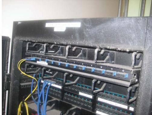
**Figure 6- Dust covered Sensitive Equipment**
